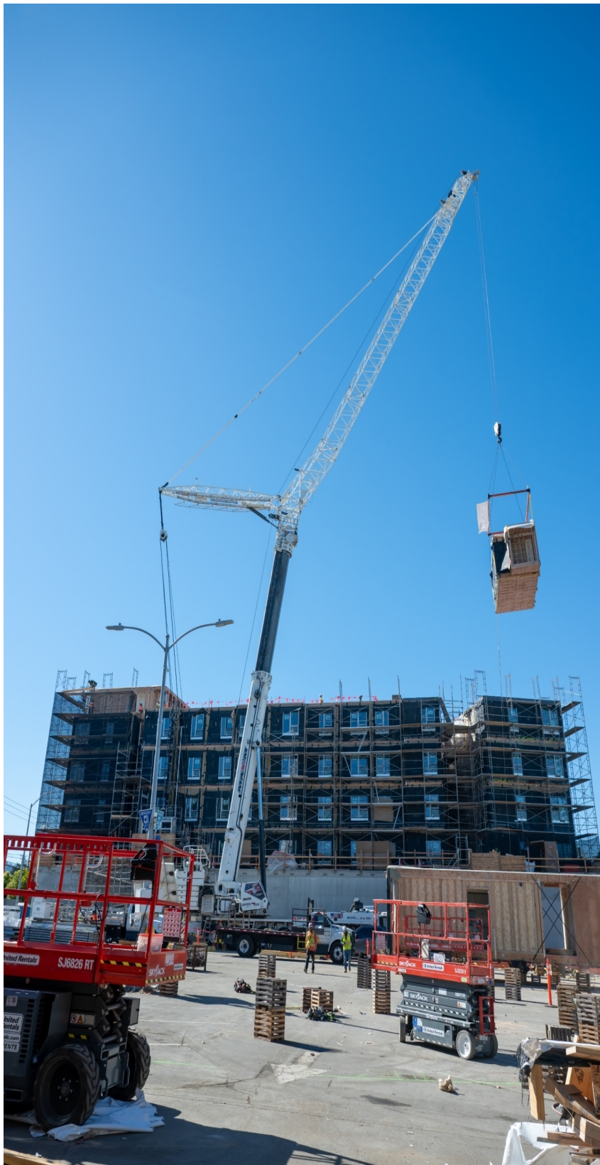
El Cerrito Plaza BART TOD, Phase I: 515 Richmond Street 70 affordable units Under Construction
