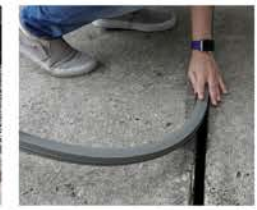
ELASTOMERIC W/ BACKER ROD FILLER
