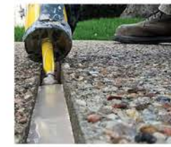
ELASTOMERIC W/ BACKER ROD FILLER
