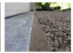
ASPHALT COLD PATCH
