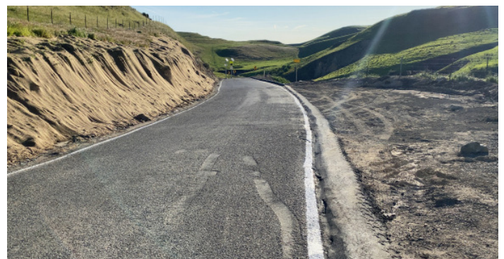
Patterson Pass Emergency Repair Completion
