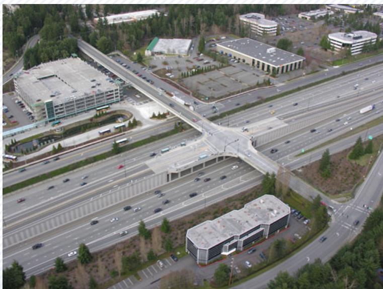
Direct access ramp, Bellevue, WA
