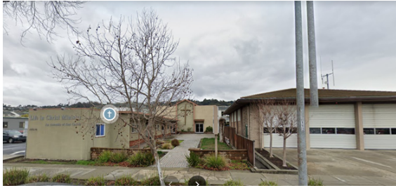
Figure 2: Property Source: City GIS.
