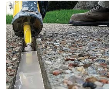
ELASTOMERIC W/ BACKER ROD FILLER
