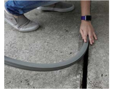
ELASTOMERIC W/ BACKER ROD FILLER
