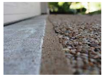
ASPHALT COLD PATCH
