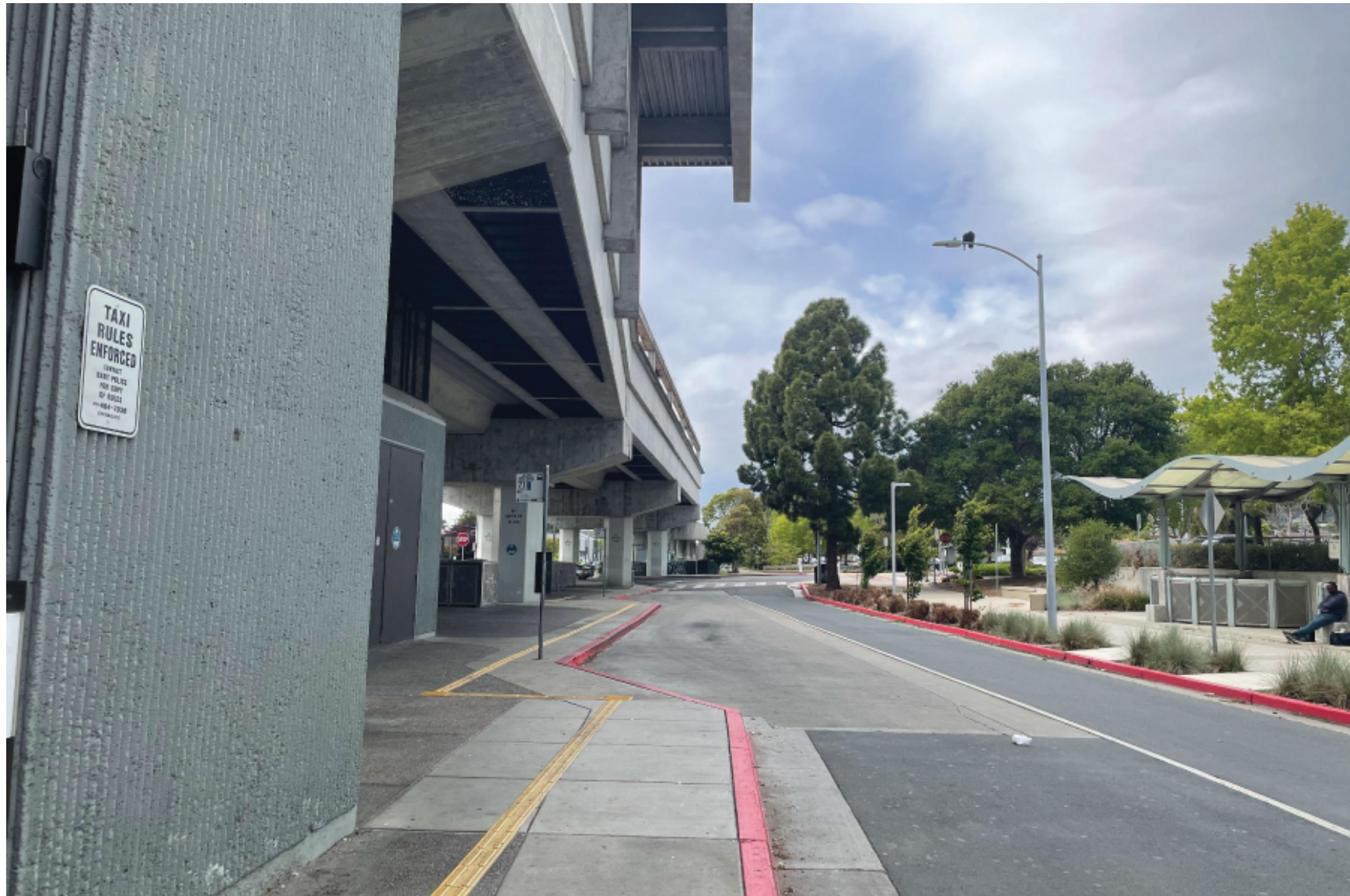
3) EAST BART STATION EXIT (LOOKING NORTH)
