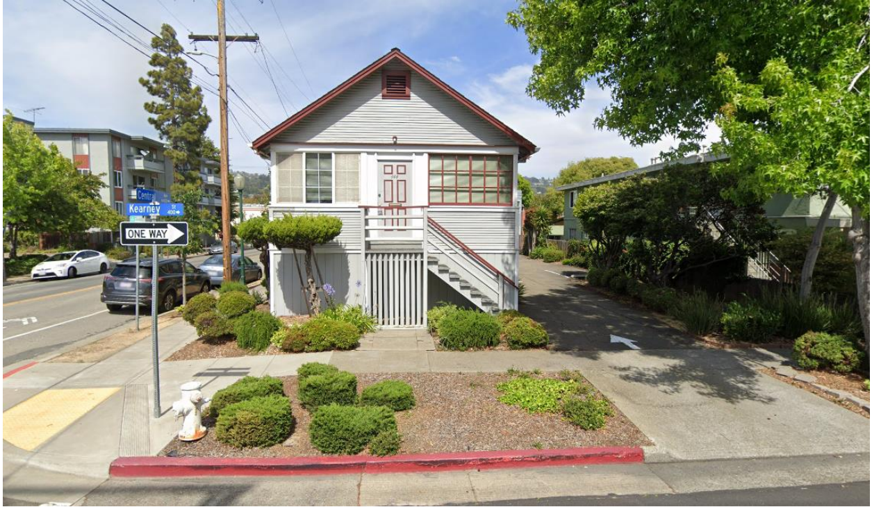
Front of the building along Kearney Street
