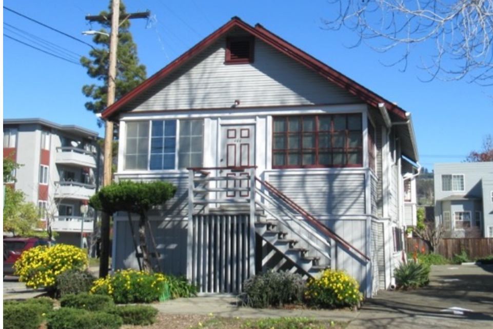
Figure 2. 444 Kearney Street, west façade, view east (Forget Me Not History, February 2022).
