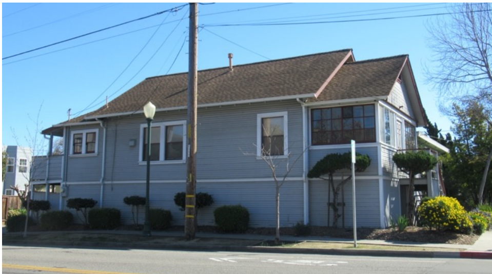
Figure 5. 444 Kearney Street, north façade, view south (Forget Me Not History, February 2022).
