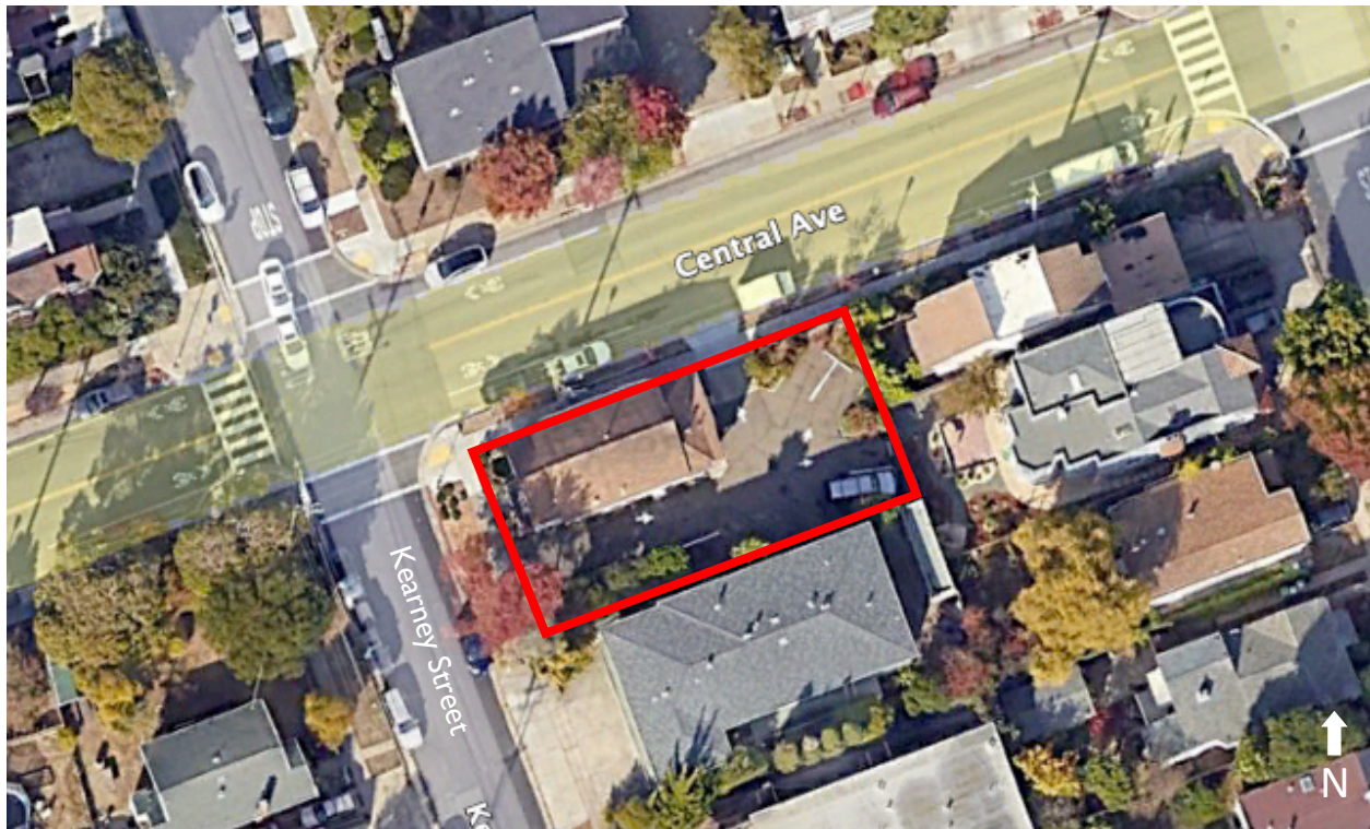
Figure 1. Aerial photograph of 444 Kearney Street (bounded in red) and immediate vicinity (Google Earth, August 2020; amended by author).
