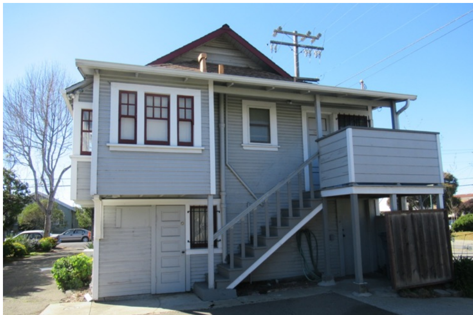
444 Kearney Street, east façade, view west (Forget Me Not History, February 2022).
