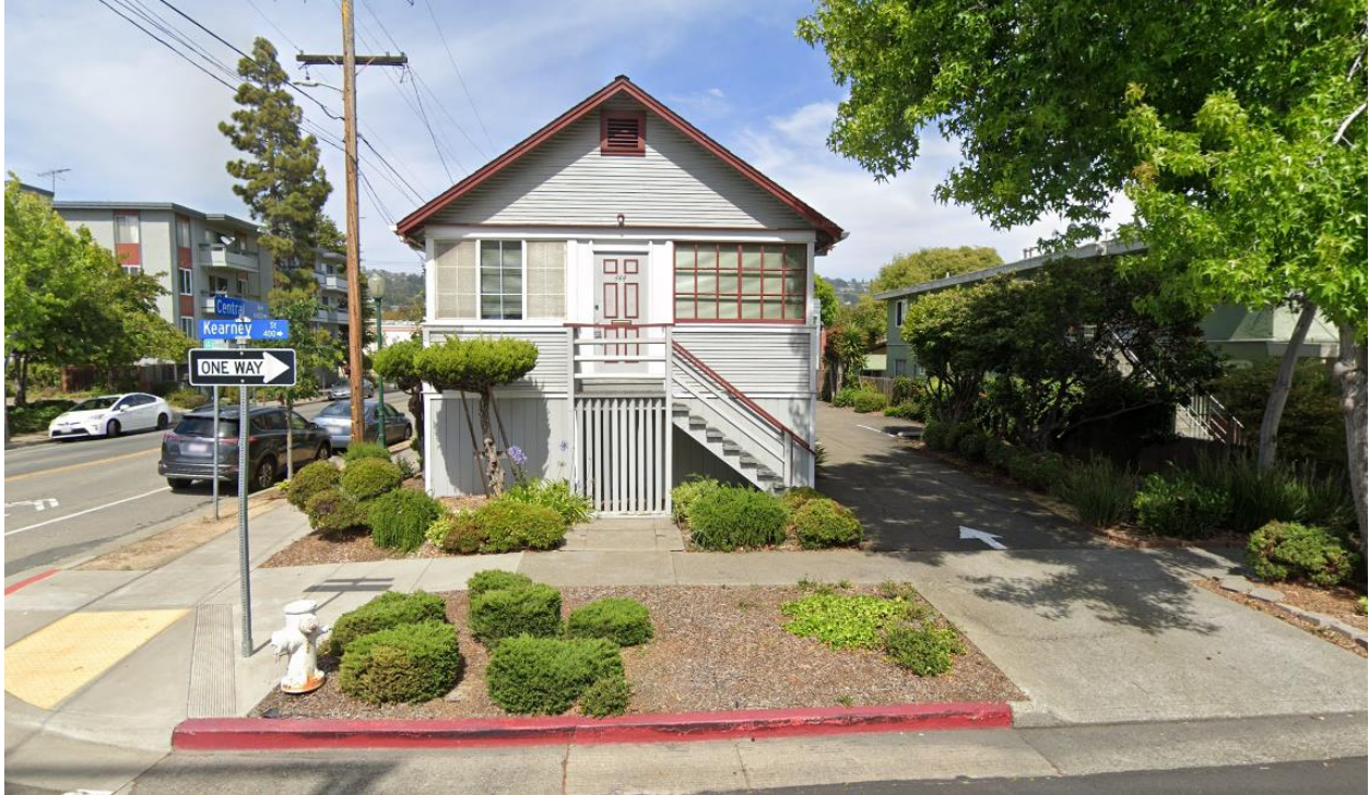
Front of the building along Kearney Street
