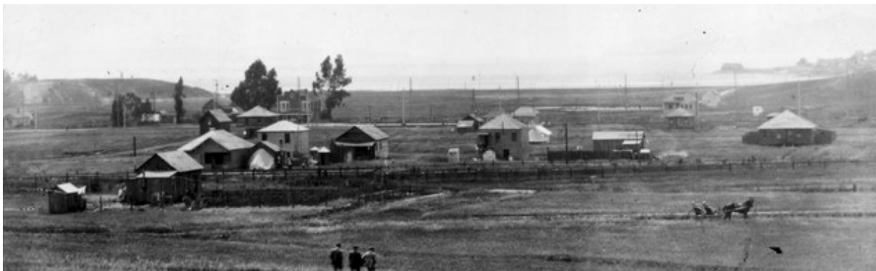
Figure 16. Early twentieth century photograph of the Henderson-Tapscott Tract No. 1 area, looking west from Richmond Avenue toward San Pablo Avenue (Contra Costa County Historical Society).
