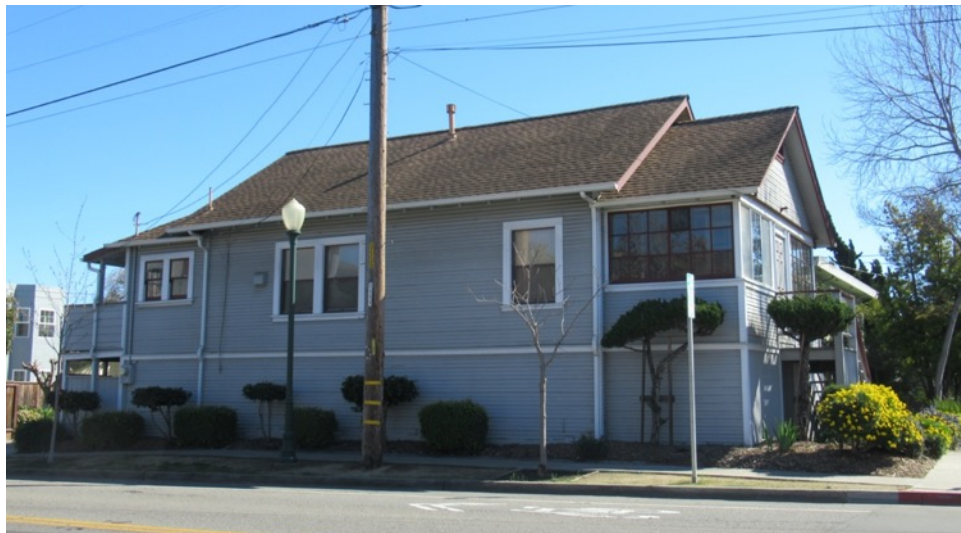
444 Kearney Street, north façade, view south (Forget Me Not History, February 2022).
