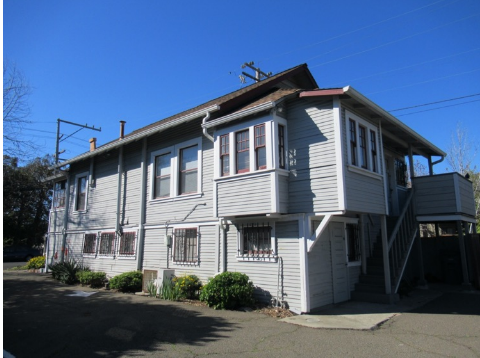
444 Kearney Street, south and east façades, view northwest (Forget Me Not History, February 2022).
