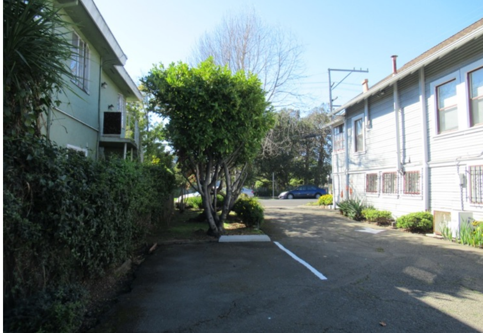
444 Kearney Street, landscaping and driveway accessing Kearney Street, view west (Forget Me Not History, February 2022).
