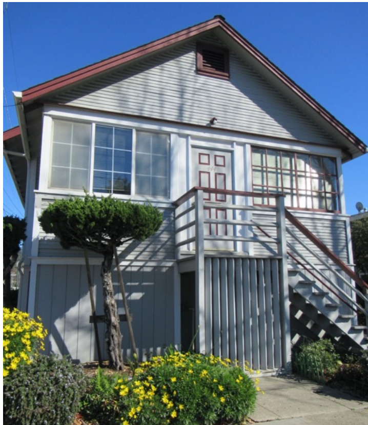
444 Kearney Street, west façade, view east (Forget Me Not History, February 2022).
