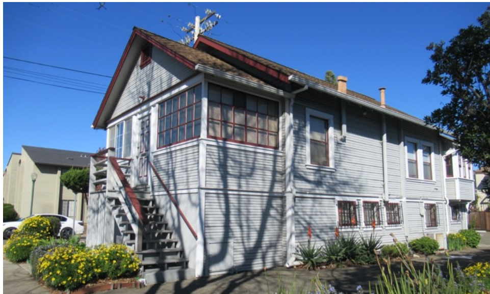
Figure 3. 444 Kearney Street, west and south façades, view north (Forget Me Not History, February 2022).
