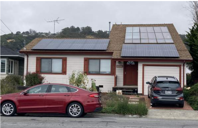
WEST (FRONT) FACADE
