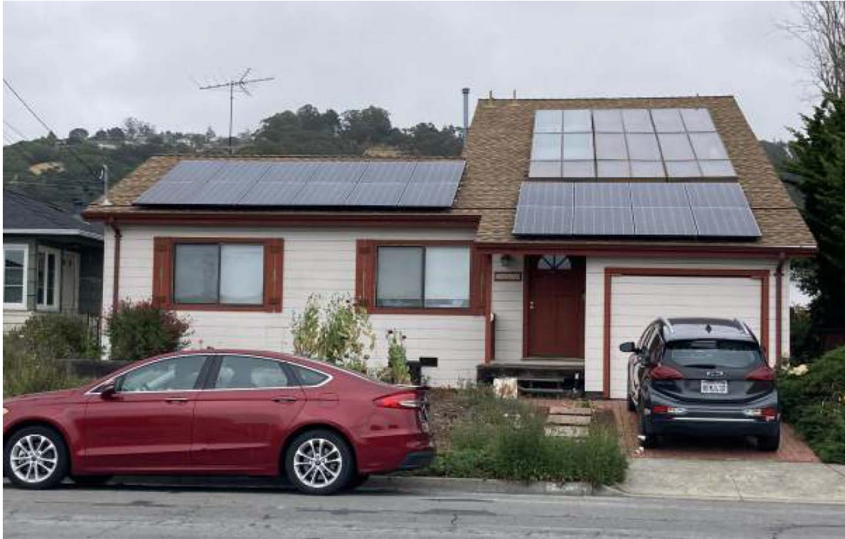
West (Front) Facade
