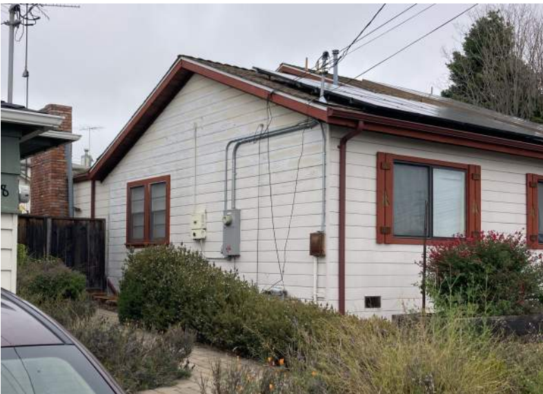
SOUTH (SIDE) FACADE
