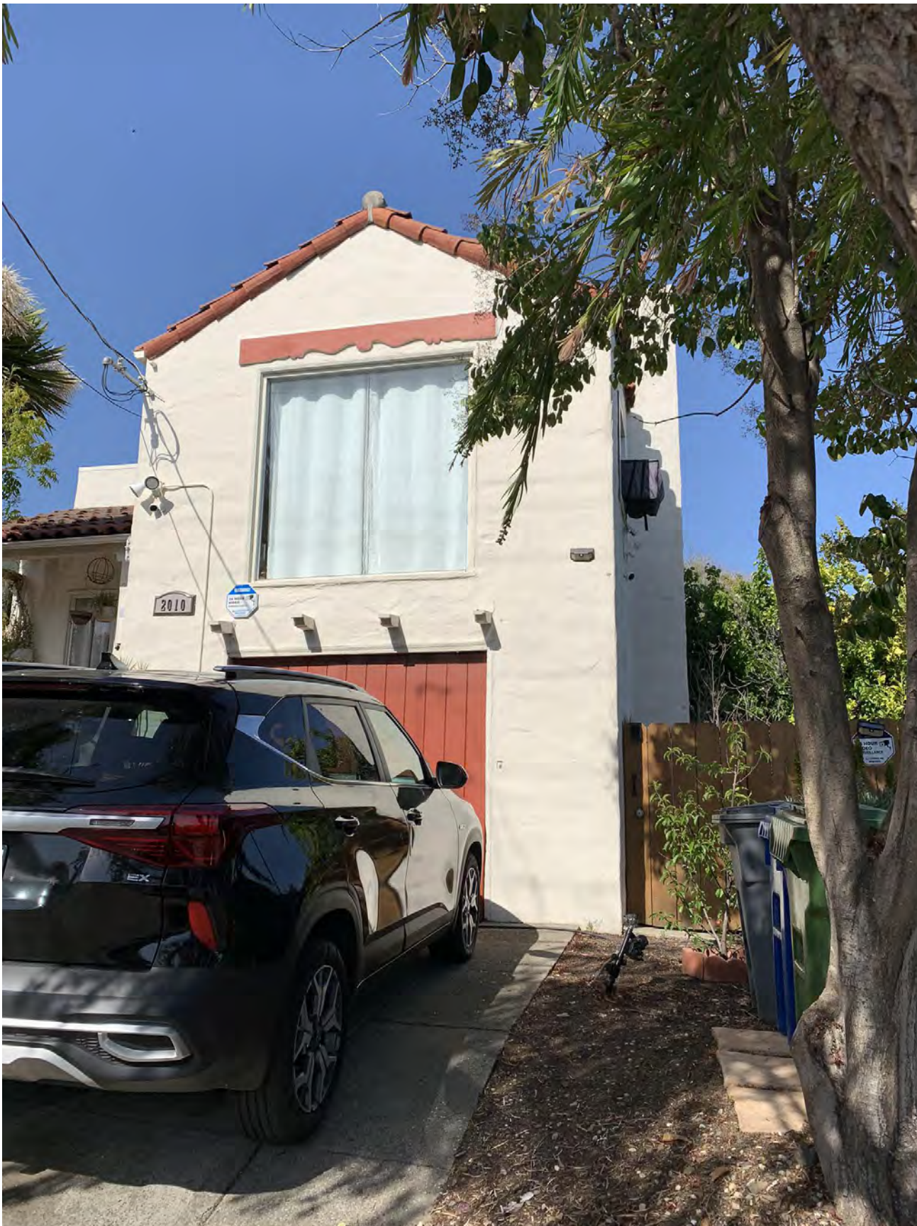
2. FRONT GARAGE FACADE
