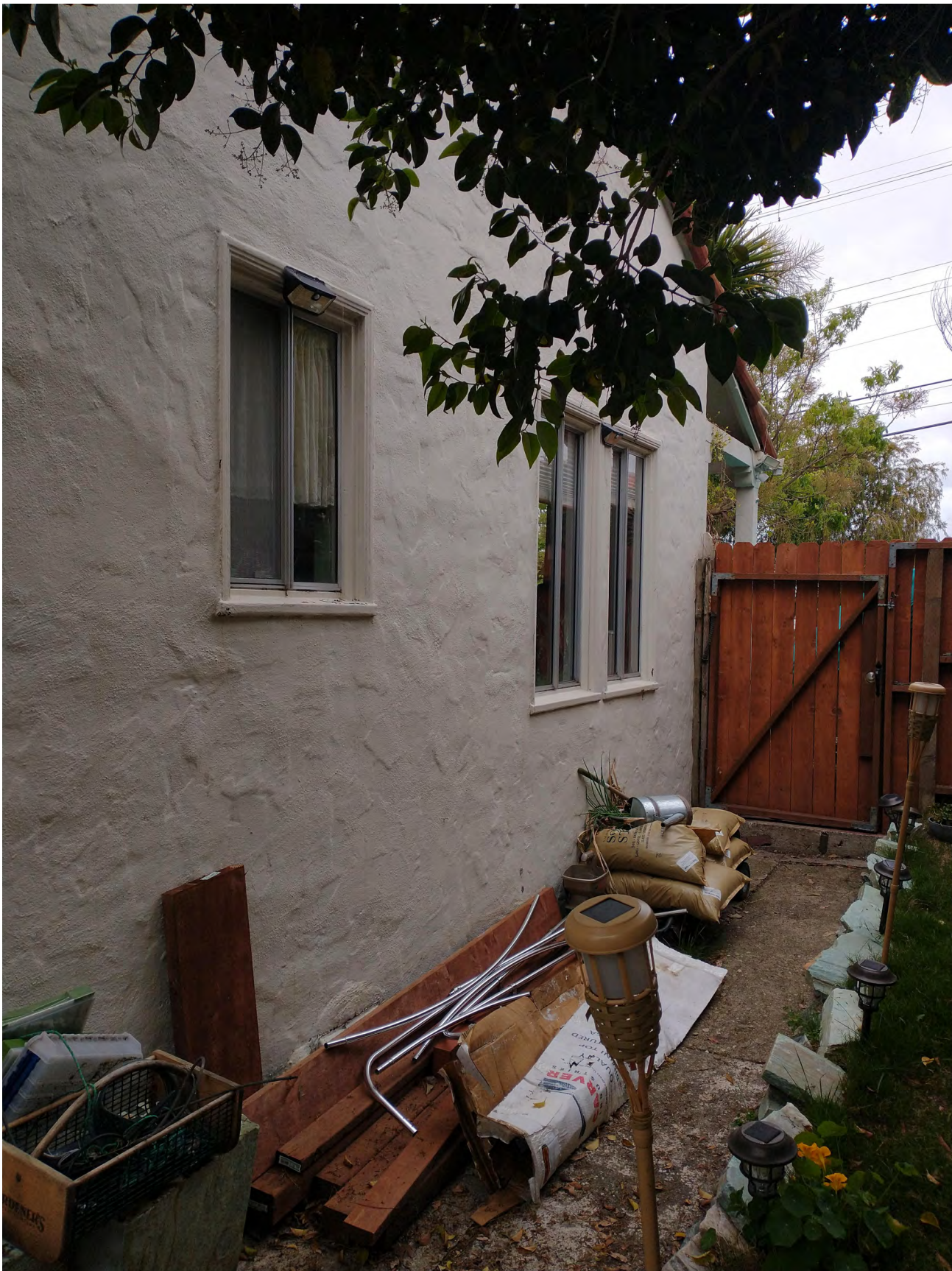
5. NORTH SIDE OF HOUSE
