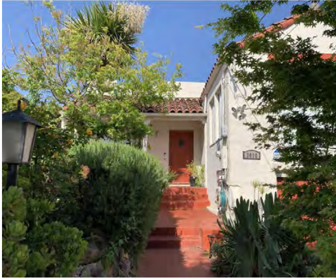
West (Front) Façade
