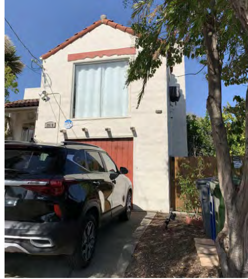
West (Front) Facade
