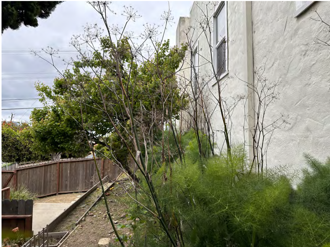
6. SOUTH SIDE OF HOUSE
