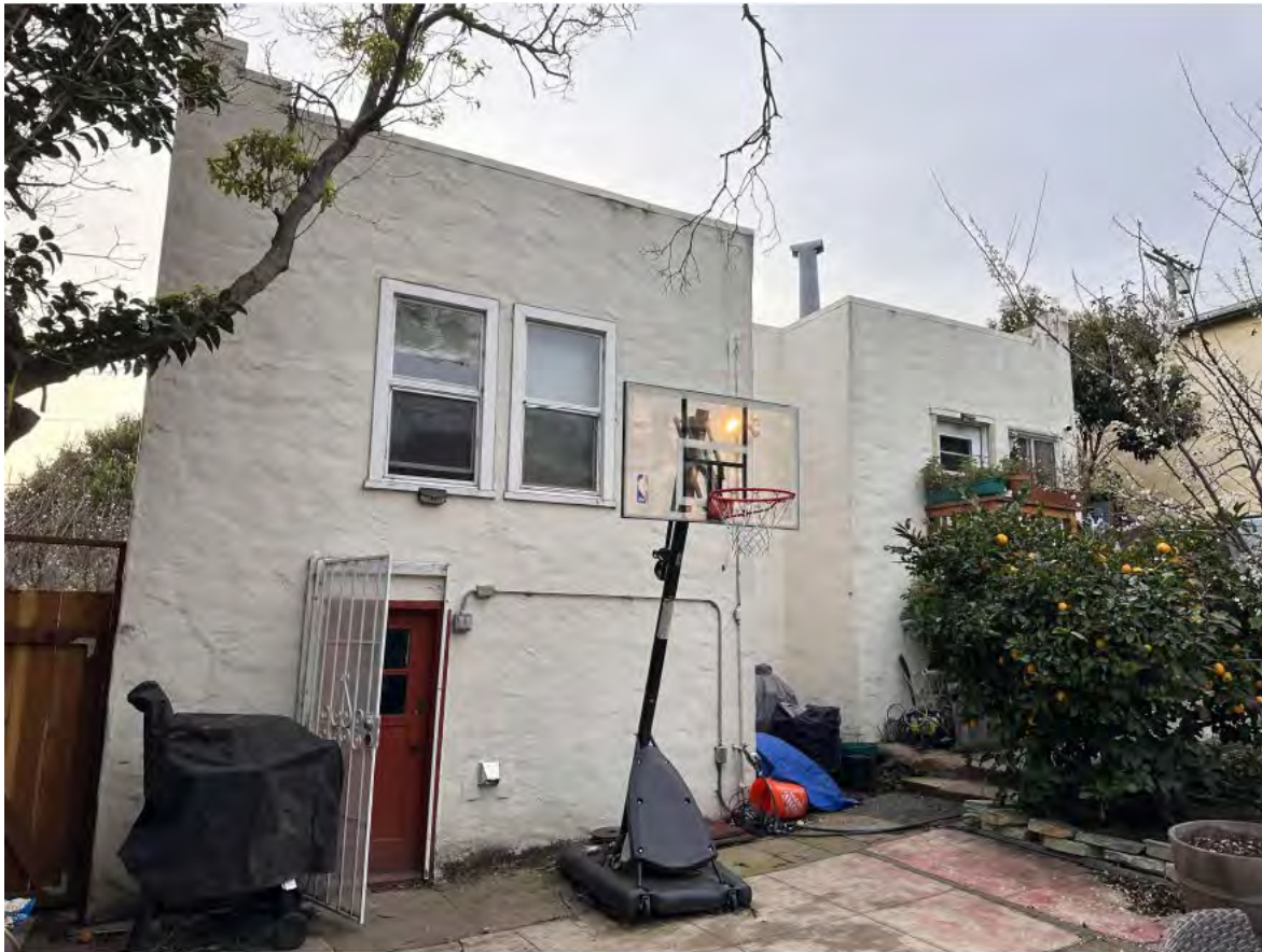
East (Rear) Facade
