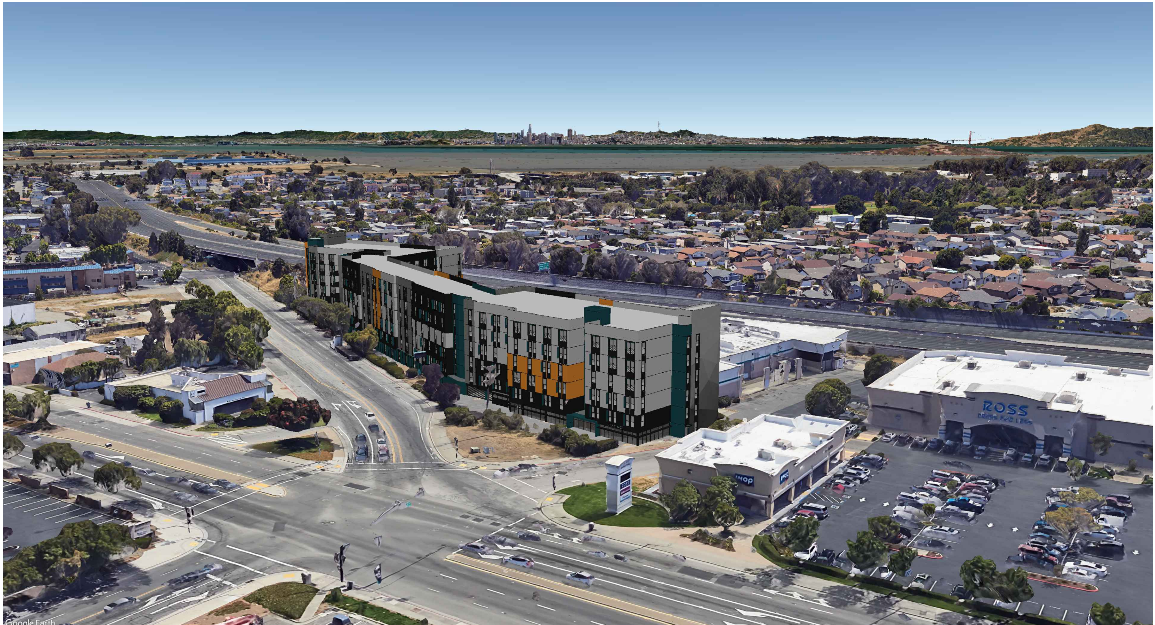
1. AERIAL VIEW LOOKING AT CORNER OF PEERLES AVE & EASTSHORE BLVD.
