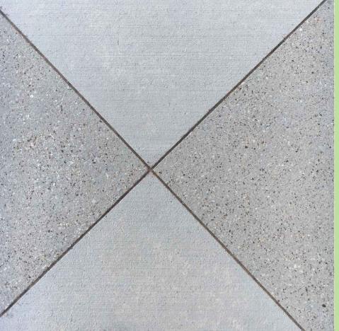
NATURAL GRAY CONCRETE IN MEDIUM BROOM FINISH AND ACID ETCH FINISH
