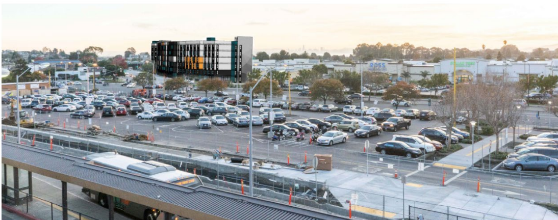
11. VIEW LOOKING SOUTH EAST FROM THE BART PLATFORM (RIGHT SIDE).
