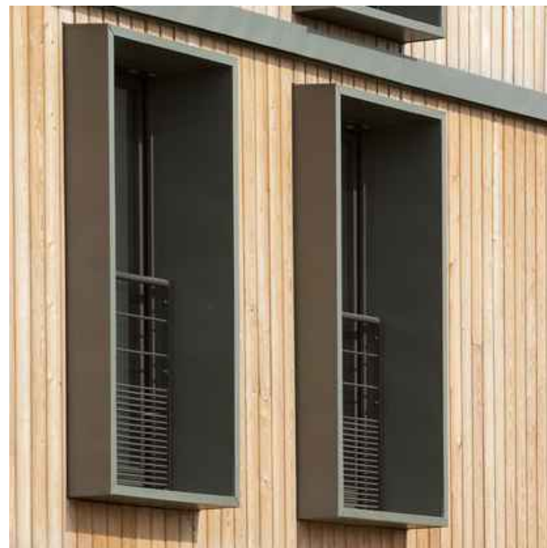
10. WINDOW EDGE WITH RAILING BLACK OR EQUAL
