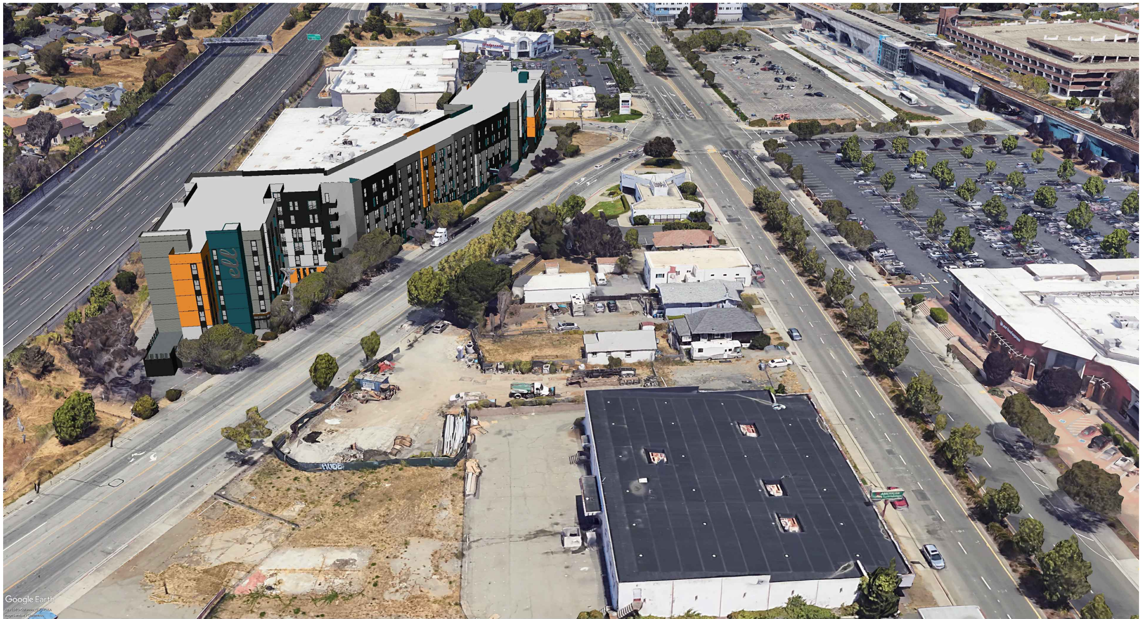
3. AERIAL VIEW LOOKING NORTH AT EASTSHORE BLVD.
