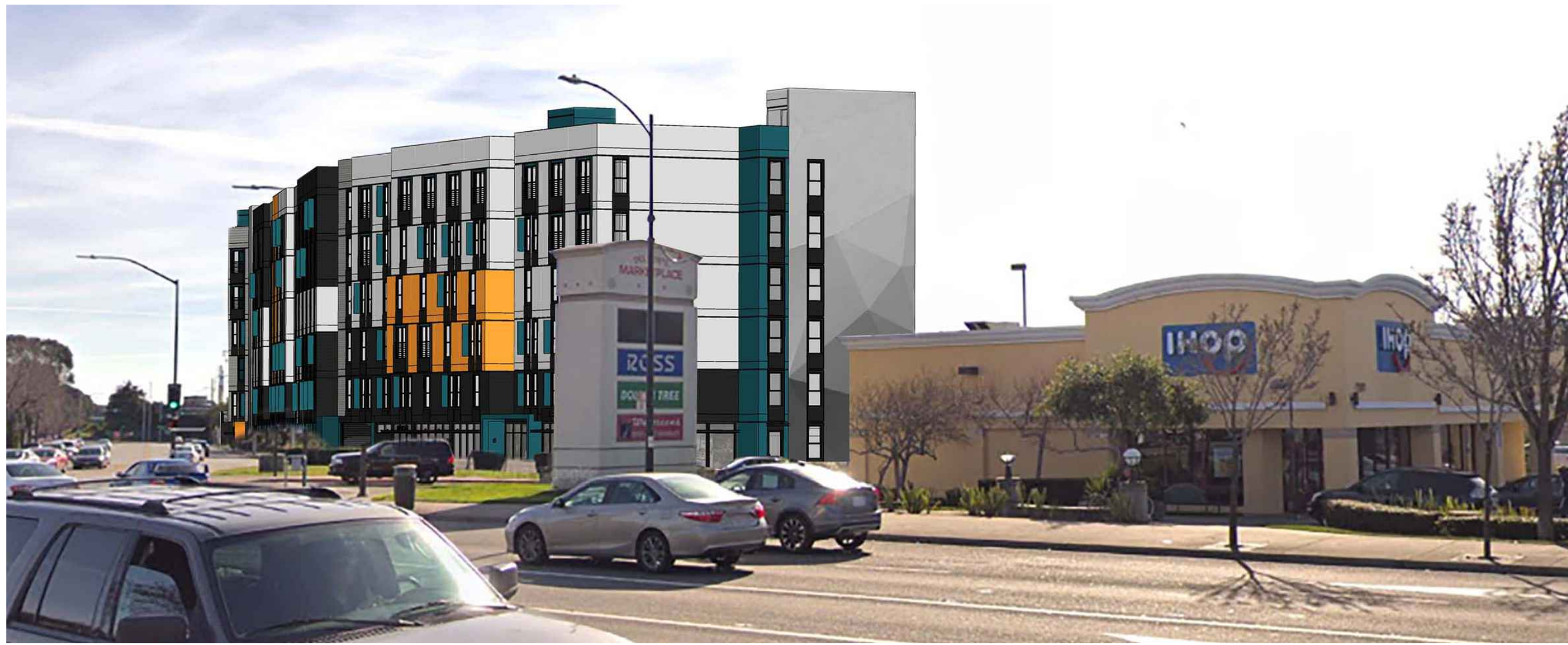
6. VIEW LOOKING SOUTHWEST ALONG SAN PABLO AVE.
