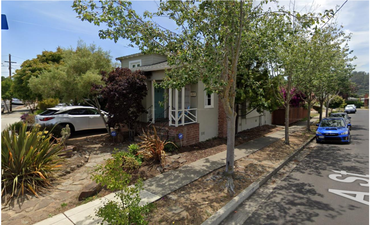
View of house from A street
