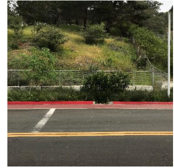
Photo: A "curb cut" in an El Cerrito rain garden, allowing stormwater to enter a landscaped area
