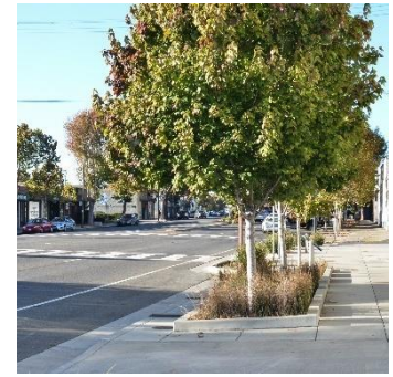
Photo: Rain garden on San Pablo Avenue in El Cerrito
