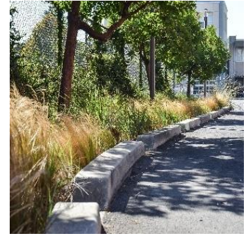
Photo: Bio-swale with "curb cuts" at the El Cerrito City Hall
