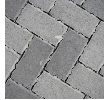
Photo: Permeable pavement, allows water to infiltrate
