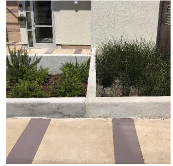
Photo: Rain gardens adjacent to a development project constructed in El Cerrito in 2018
