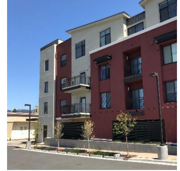
Photo: Rain gardens outside of a new development project, completed in 2018
