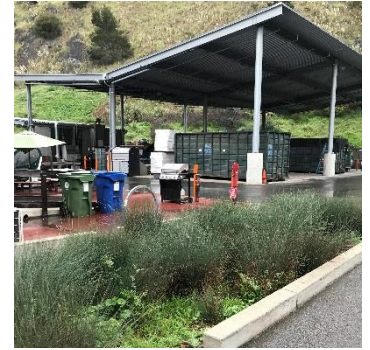
Photo: Rain garden and rain water harvesting roof at the El Cerrito Recycling Center
