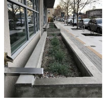
Photo: Rain garden adjacent to a development project on San Pablo Avenue in El Cerrito
