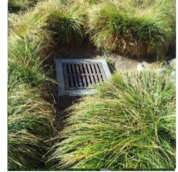
Photo: Storm drain inlet inside bio-swale
