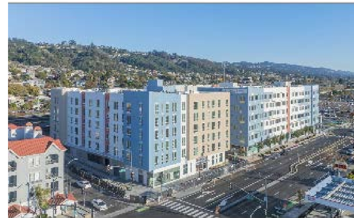
Mayfair Station + Elora (2026): 156 market-rate units, 69 affordable units, and 4 new ground-floor businesses under construction
