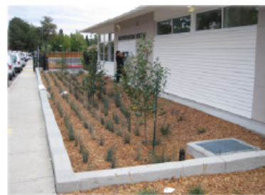
Bioretention facilities should be designed so the surface reservoir floods evenly to the design depth. This facility provides stormwater treatment and flow duration control for a Pittsburg office building and parking lot.
