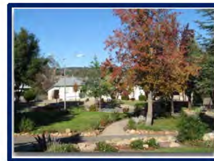
Marsh Creek Detention Facility
