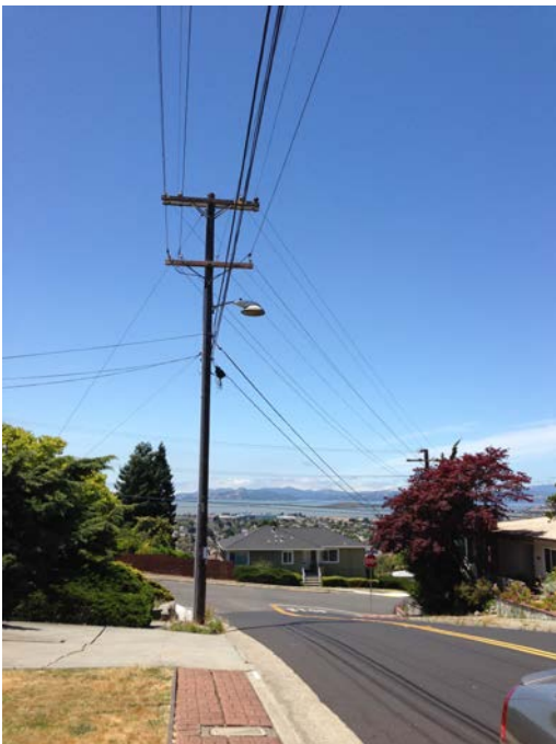
Existing utility pole near 7800 Eureka Avenue.
