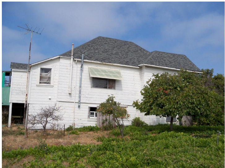
Figure 11. South façade Source: Christopher VerPlanck
