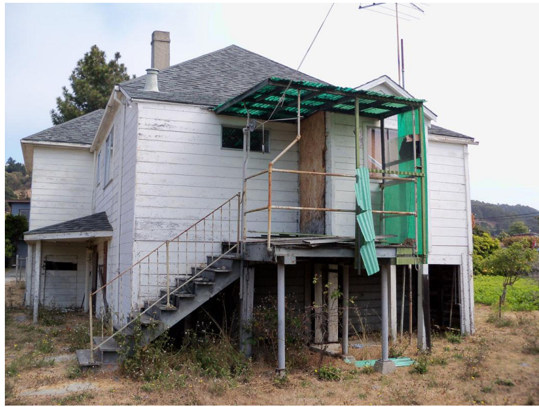
Figure 10. Rear (west) façade Source: Christopher VerPlanck
