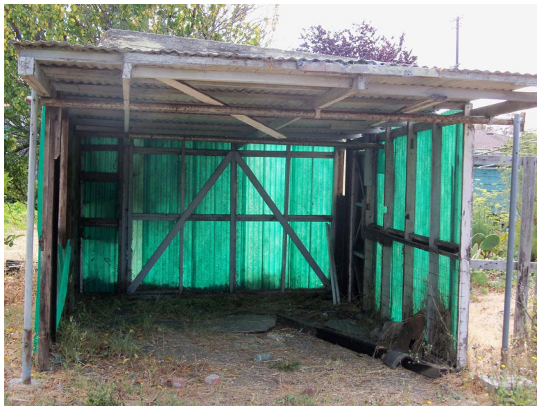
Figure 13. Shed; view toward south
