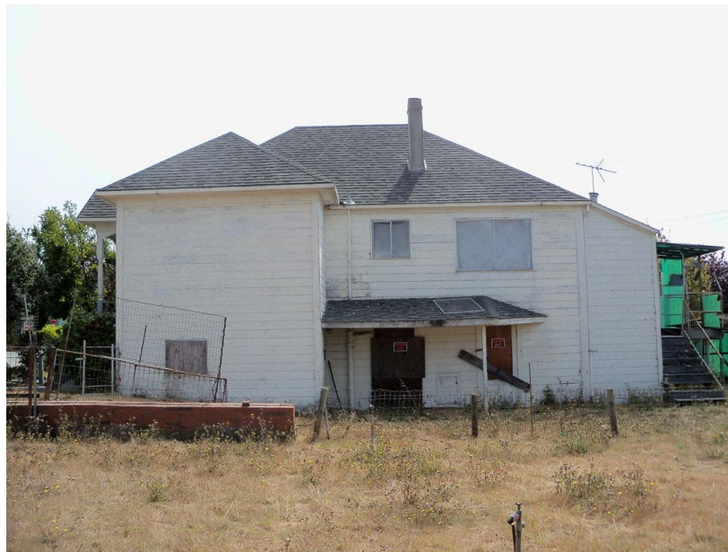
Figure 9. North façade Source: Christopher VerPlanck
