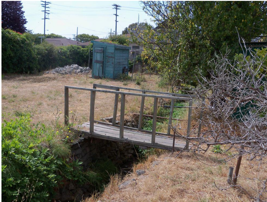
Figure 15. Creek and bridge, looking southwest Source: Christopher VerPlanck
