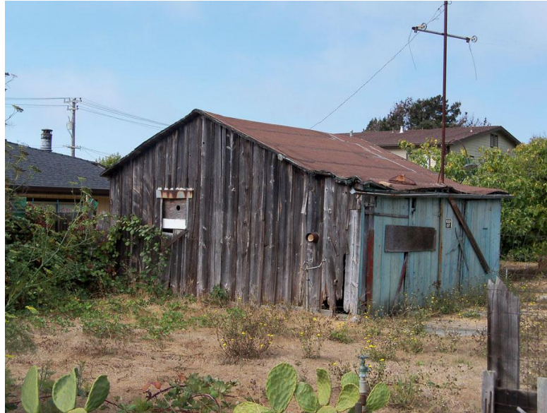
Figure 12. Garage; view toward north Source: Christopher VerPlanck
