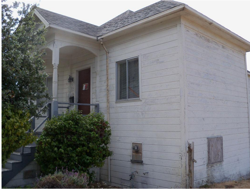
Figure 8. Right bay of primary façade Source: Christopher VerPlanck
