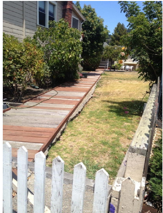
Figure 4: Wooden Lid Culvert on Downstream Parcel
