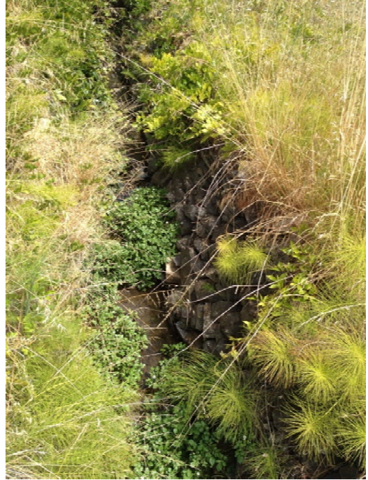
Figure 2: Existing "U" Shaped Channel
