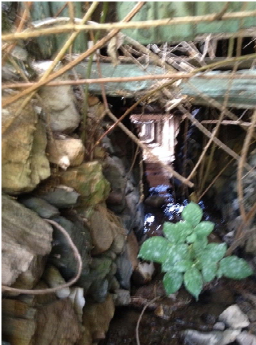
Figure 3: View Looking into Downstream Culvert
