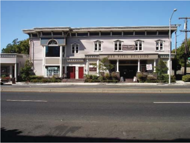
The Vital Building (formerly the Historical El Cerrito Mill & Lumber Building). The building is a perfect fit for shallow lot sizes, abutting single-family homes. 10837 San Pablo at Orchard Ave., Richmond Annex Building height: 25 ft. as verified with City records.
