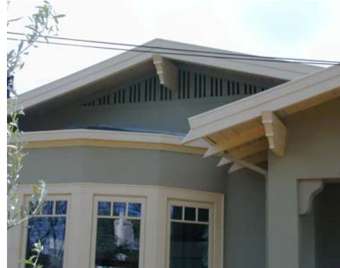
Vents as an architectural element
