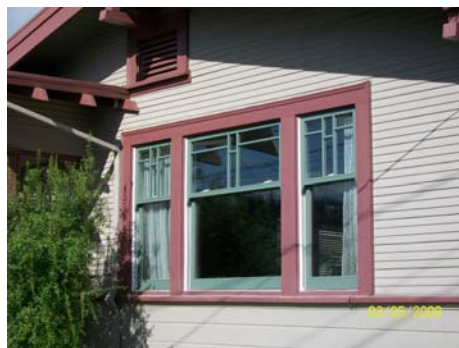
2" window recess from face of wall
