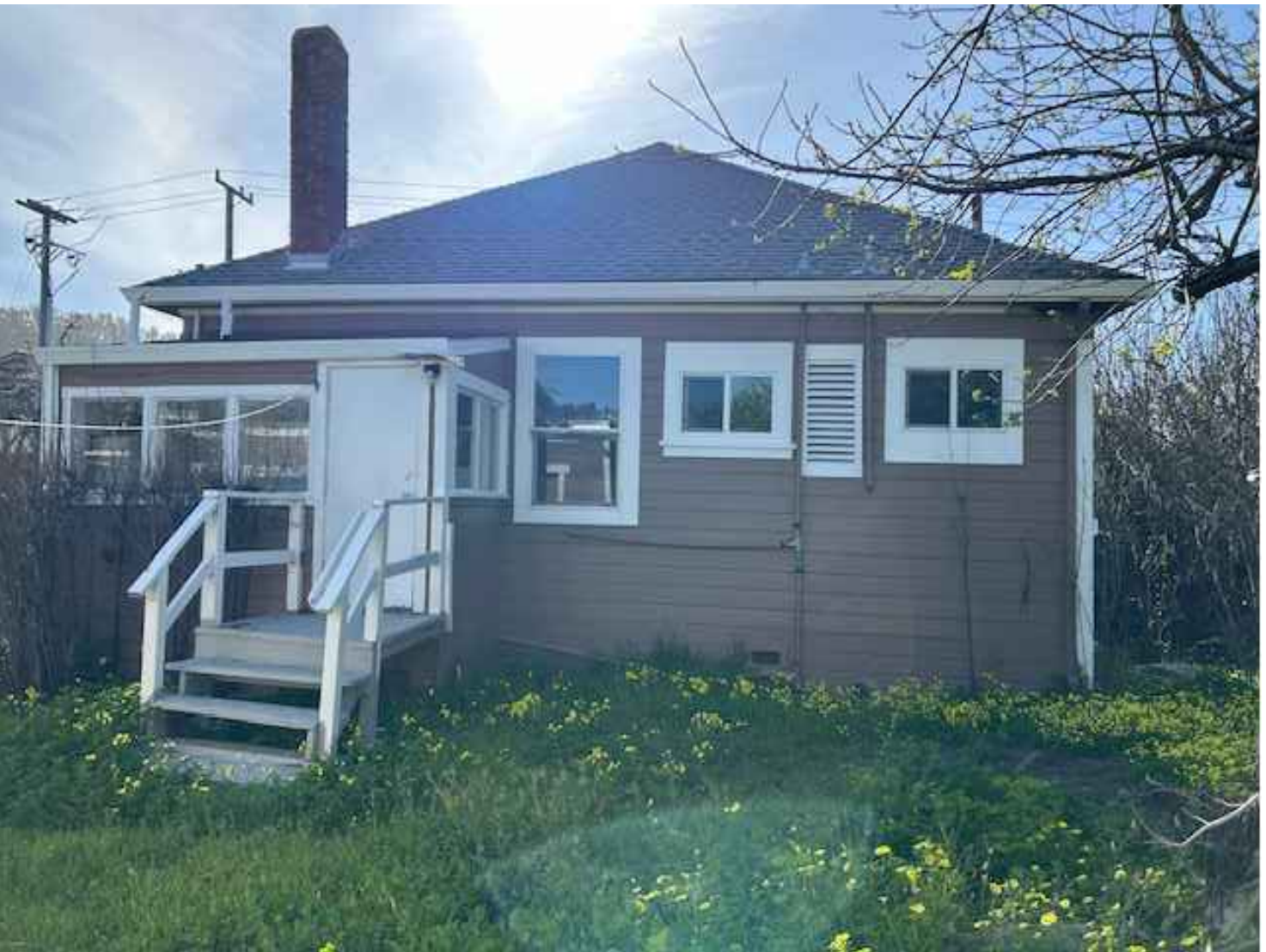
J. REAR YARD VIEW OF EXISTING HOUSE AT 412 LEXINGTON AVE - STRUCTURE TO BE DEMOLISHED
