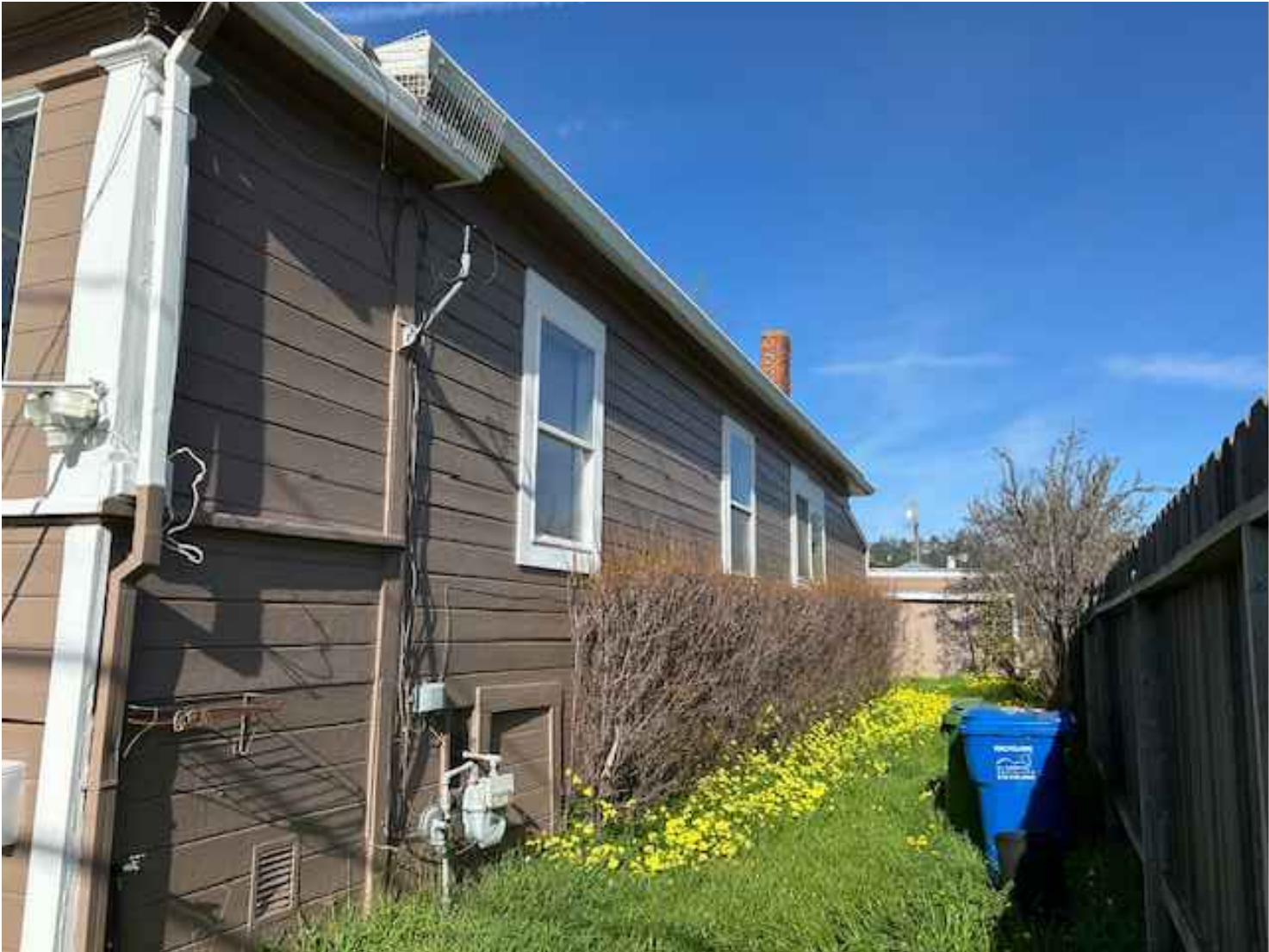
H. SIDE YARD (SOUTH) VIEW OF 412 LEXINGTON AVE - STRUCTURE TO BE DEMOLISHED
