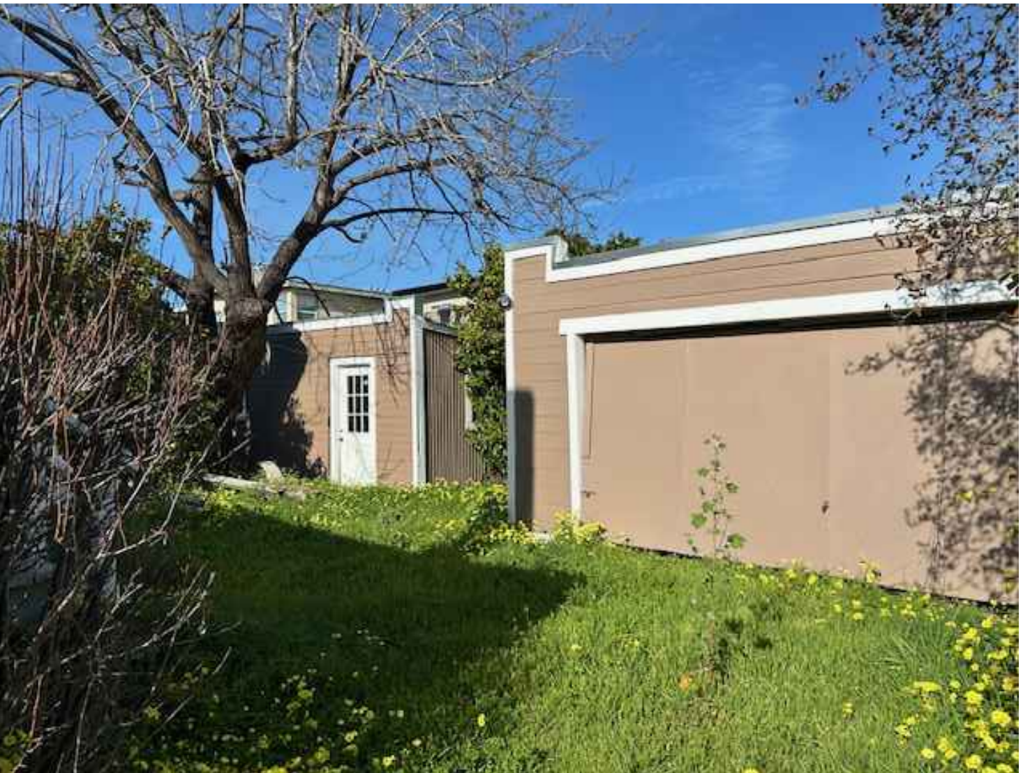
I. BACK YARD VIEW OF GARAGE AND SHED AT 412 LEXINGTON AVE - STRUCTURE TO BE DEMOLISHED
