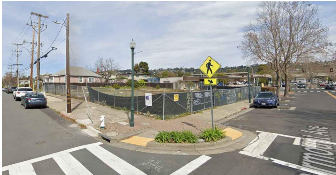
Southwest corner of the site - Existing Conditions
