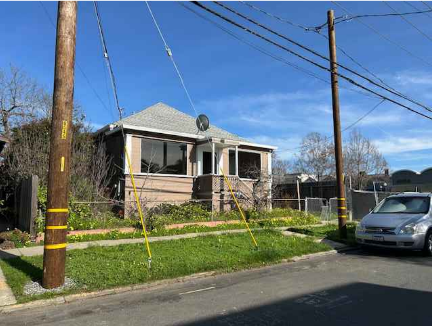
G. STREET VIEW OF 412 LEXINGTON AVE - STRUCTURE TO BE DEMOLISHED
