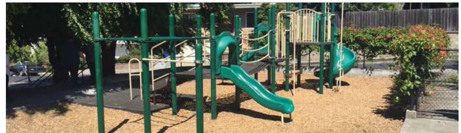
FIGURE 30. PLAYGROUND AT POINSETT PARK, IN 'GOOD' CONDITION
